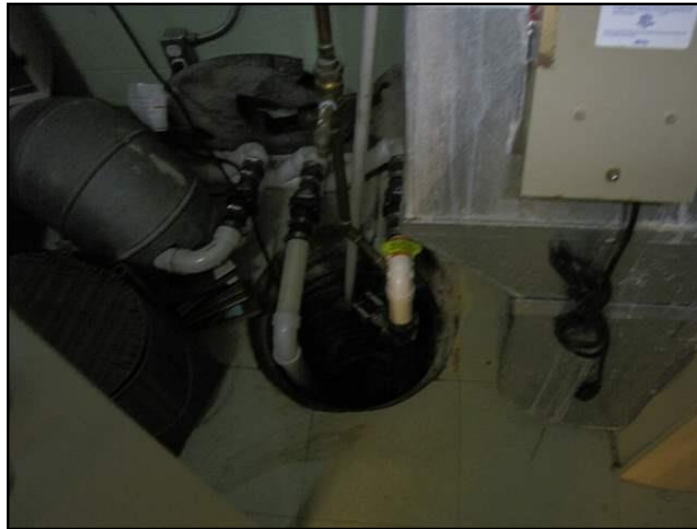
135. Back up sump pump: Siphon Jet
