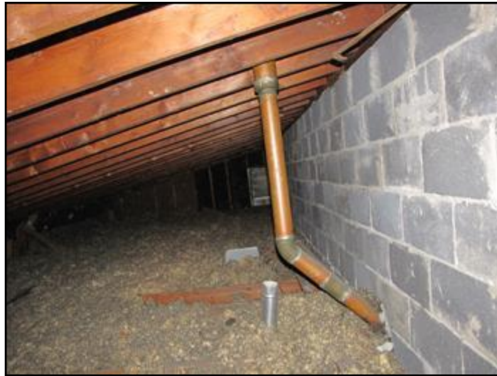
190. Poor termination location
