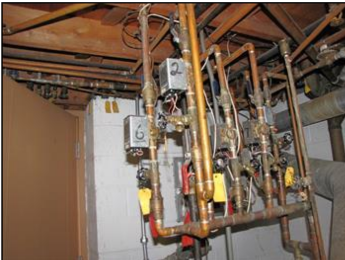
60. Hot water radiant heat
