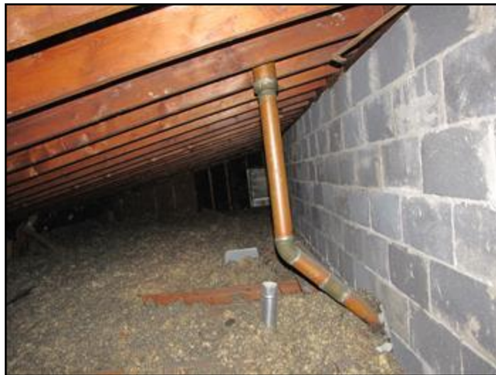
12. Poor termination location
